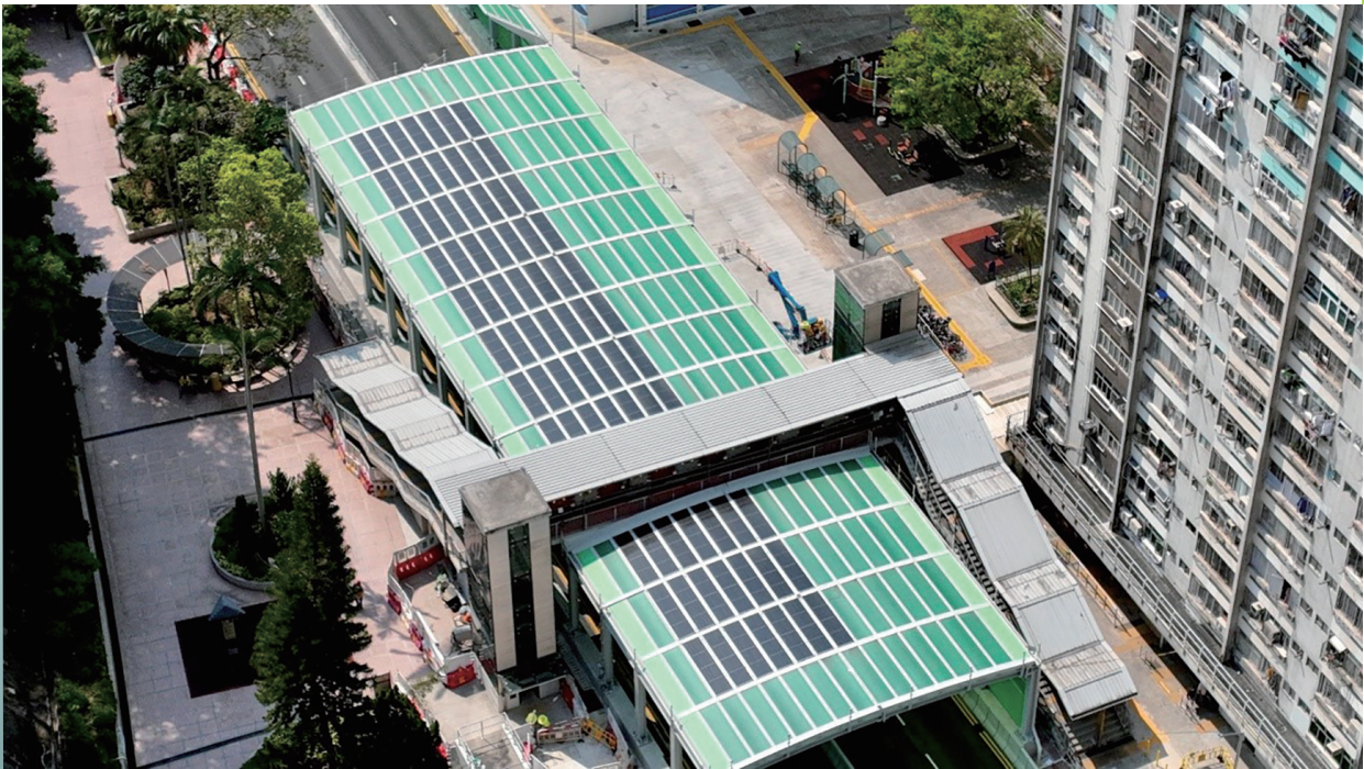
BIPV photovoltaic integrated soundproofing screen is applied in the project of "Widening the Castle Peak Road between Kwun Tsing Road and Hai Wing Road"
